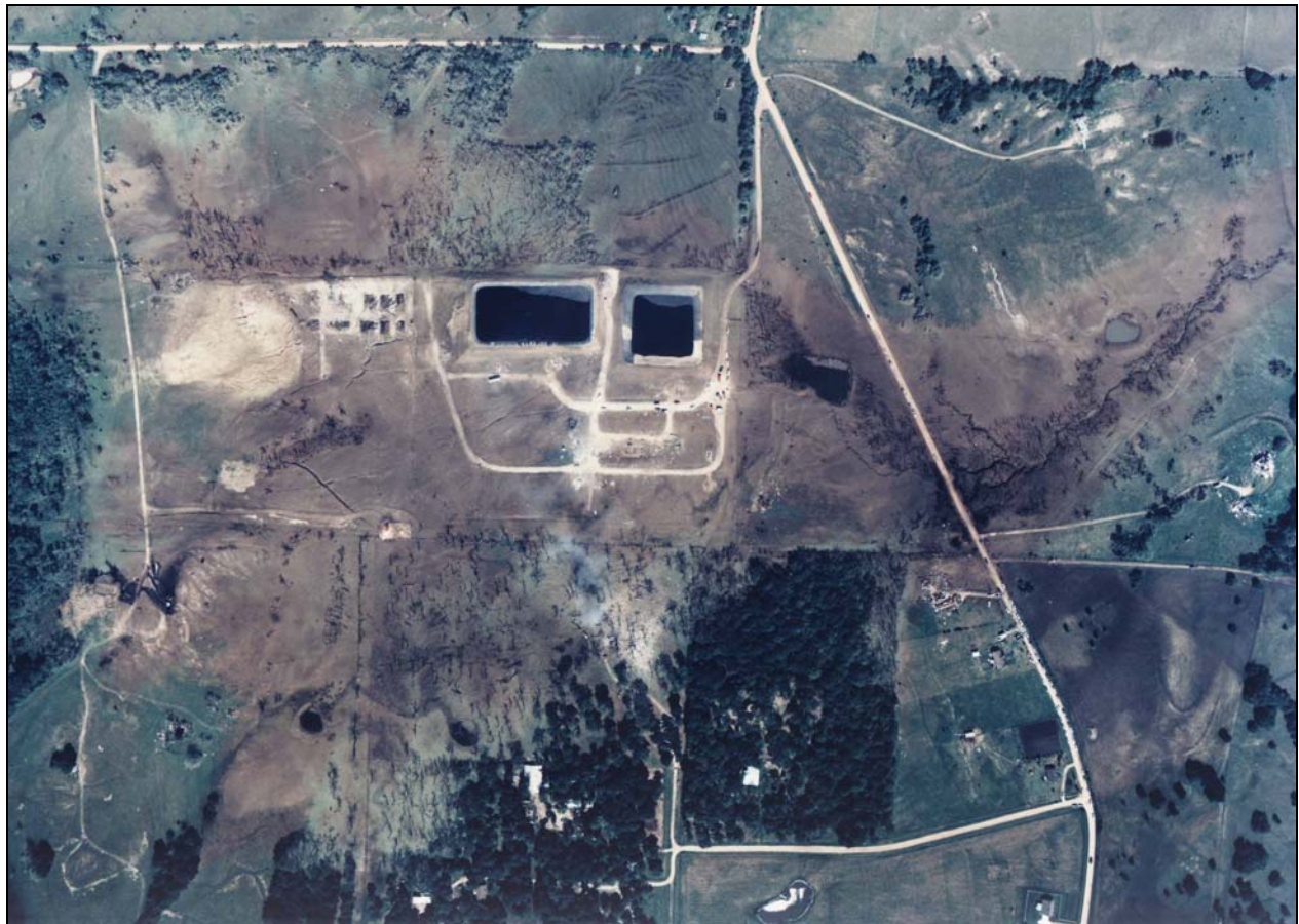
Figure 1: Aerial View After the Brenham Gas Explosion
